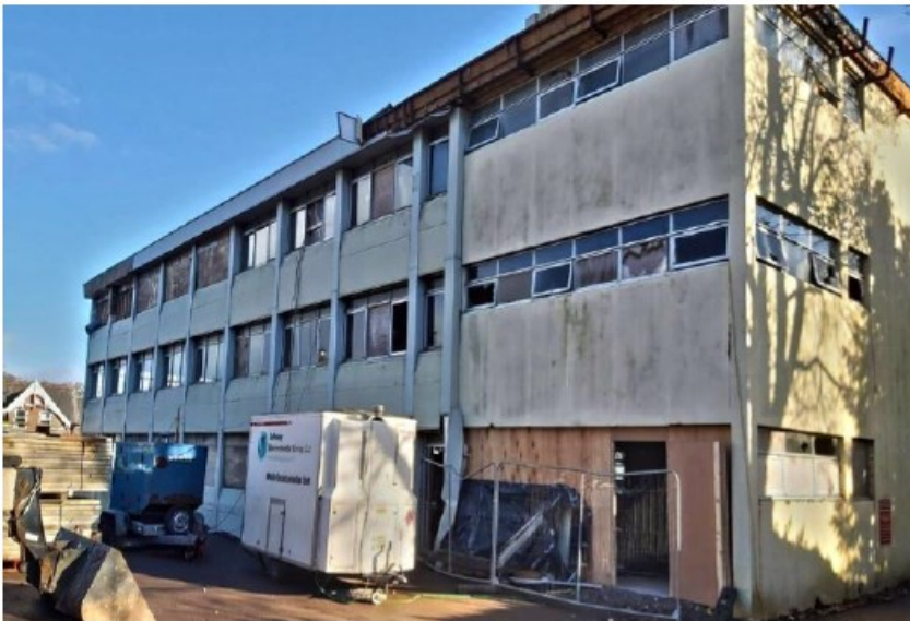
Springville House before the office-to-residential conversion
